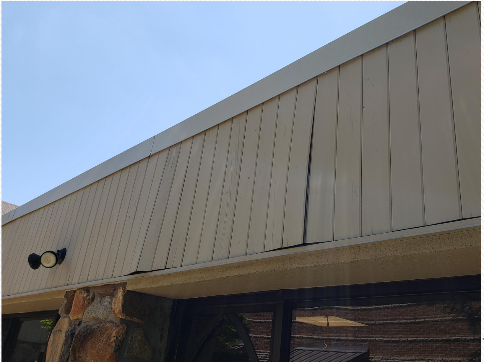
cog roof trim replacement
